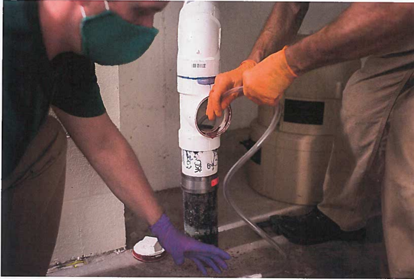
A system at U.N.C. Charlotte will automatically take wastewater samples from residence hall basements. Pete Kiehart for The New York Times
