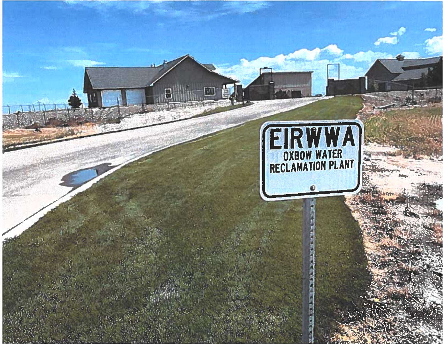
The Oxbow Treatment Plant in Bingham County. | Andrea Olson, EastIdahoNews.com
